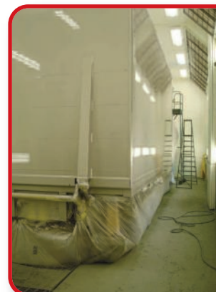
Below: Renault Trucks South paint shop
